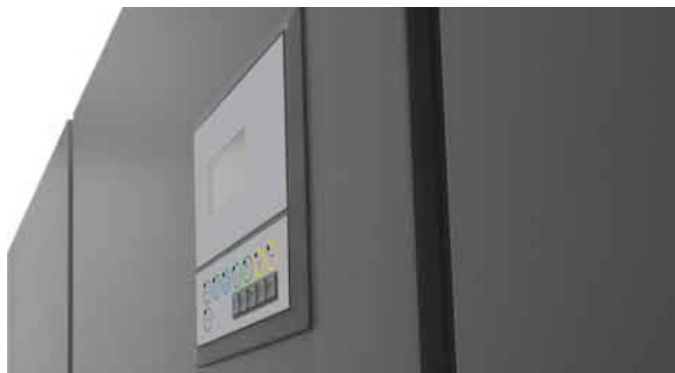
Modulating controller display and keypad
