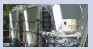
The YVWA chiller can efficiently handle the high condenser pressure required for dry cooling.
